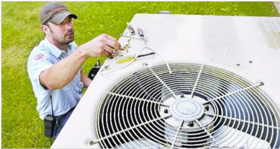
Larry Dudding, a service technician with Kennedy's Inc., cleans and checks a furnace/air conditioner unit Friday at a Van Buren home. jmorehead@chronicle-tribune.com
